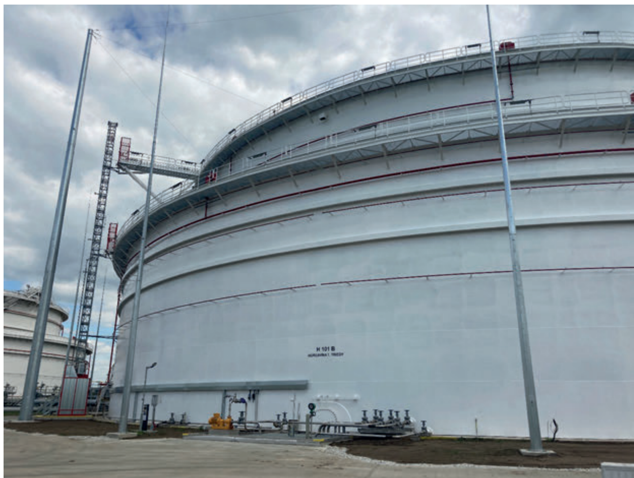
Image 2: Oil tank no. H101B in PS 4 Tupá
